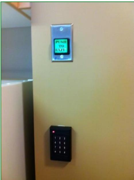
*This is an example of a keypad entry/exit system inside a unit for parolees with residency conditions. The keypad is connected to a computerized system which can be monitored by staff, and also has an emergency exit button in the event of a crisis which dispatches emergency response and unlocks the unit without a key code.*
